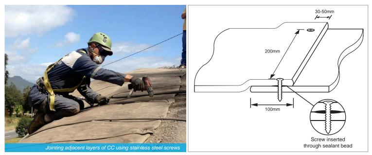
If a higher level of impermeability is required (for example on an outfall) then a bead of sealant such as Clearfix can be applied in the overlap prior to screwing. If screws are not suitable (for example if laying on a geomembrane) then an adhesive sealant such as Clearfix or a concrete mortar joint may be used.
