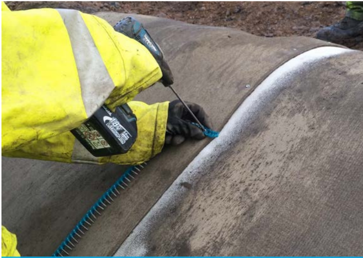
Transverse layers with a 100mm overlap were screwed in place
