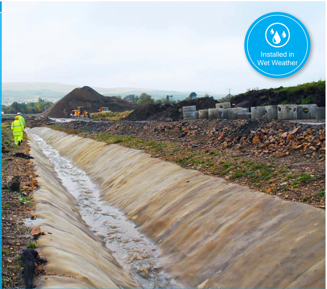
A completed section of ditch
