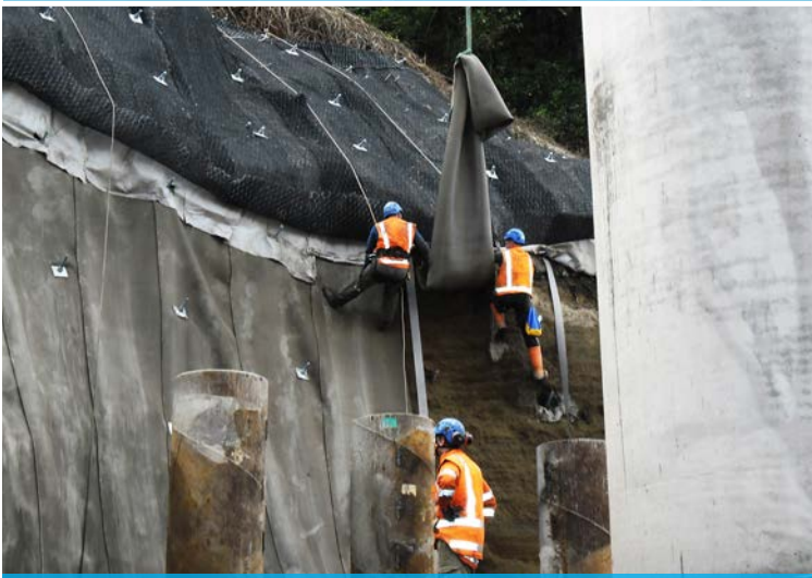
Installation under the geotextile
