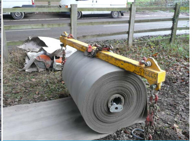
Bulk roll and spreader beam
