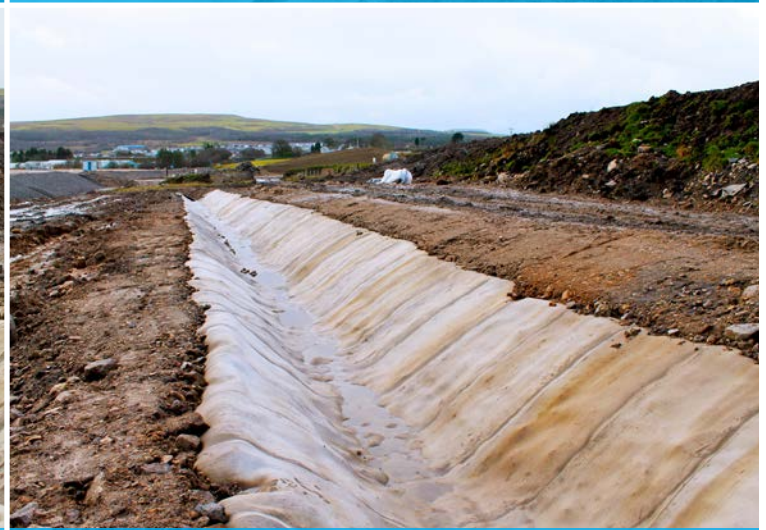
The finished ditch
