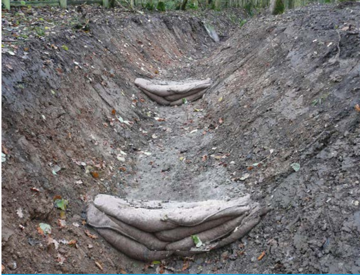
Concrete sandbag cascades
