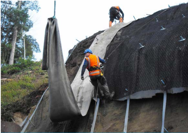
Engineering anchors pushed through the matting
