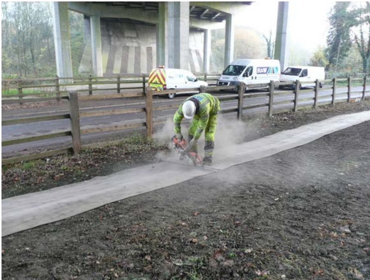
Cutting CC to length on site
