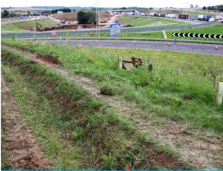
Site prior to works
