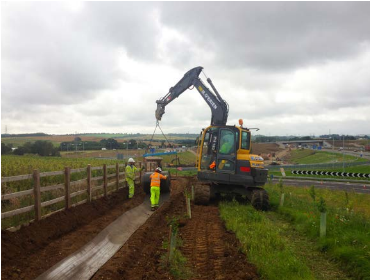
Deployment of CC via spreader beam
