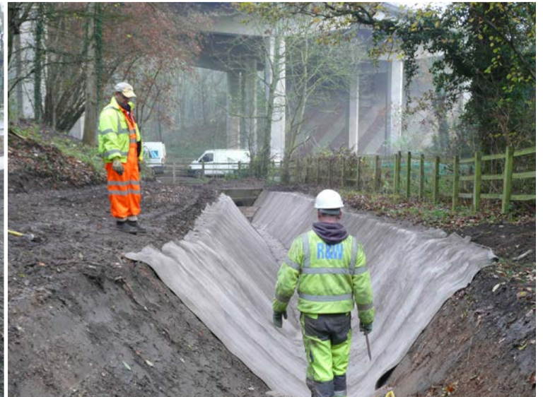
Pegging into the crest
