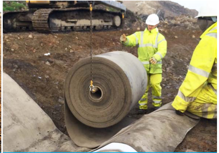
Plant was used to unroll and place the material
