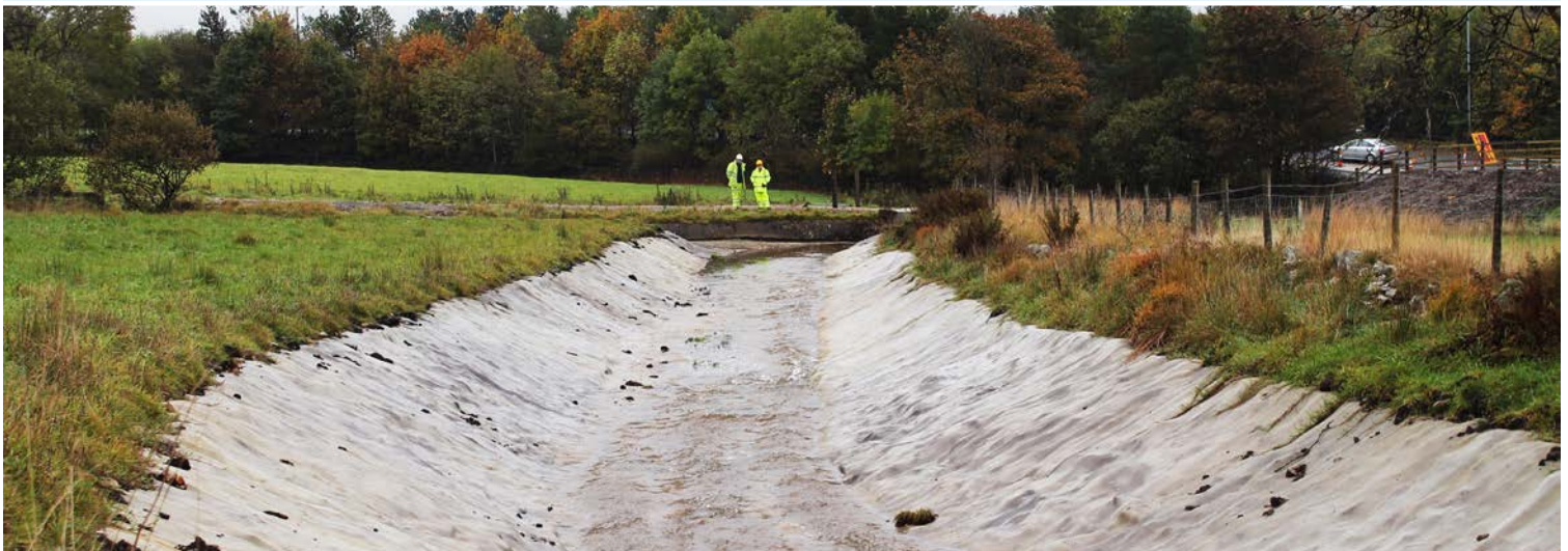
A completed section of ditch
