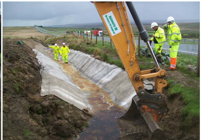
Allowing the live water course to help hydrate the CC
