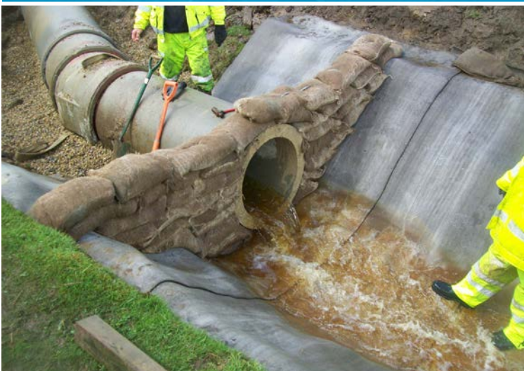
Concrete sandbag header constructed on top of the CC
