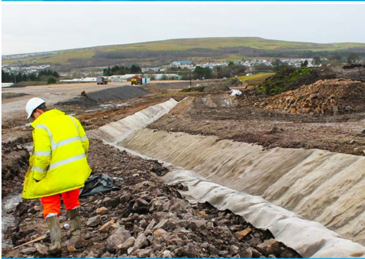
Transverse layers backfilled into the anchor trench along crest
