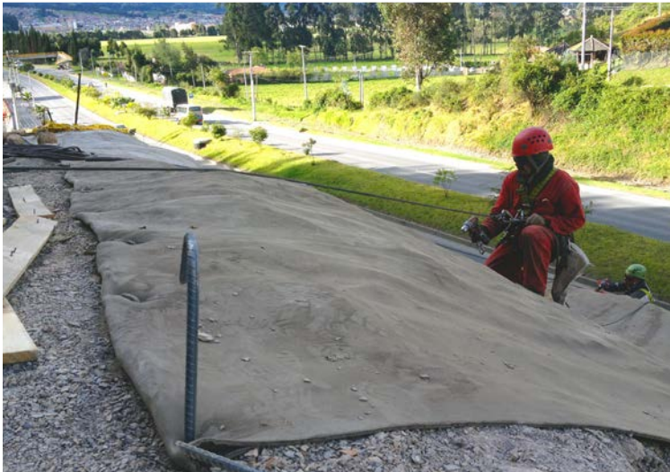
CC was fixed to the top of the slope using steel ground pegs
