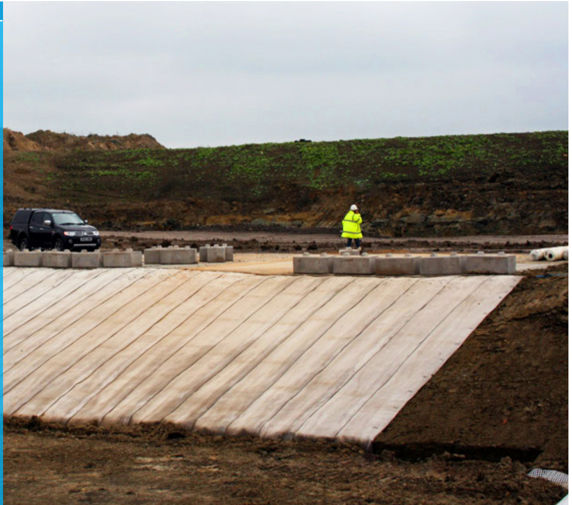
Bank protection installation
