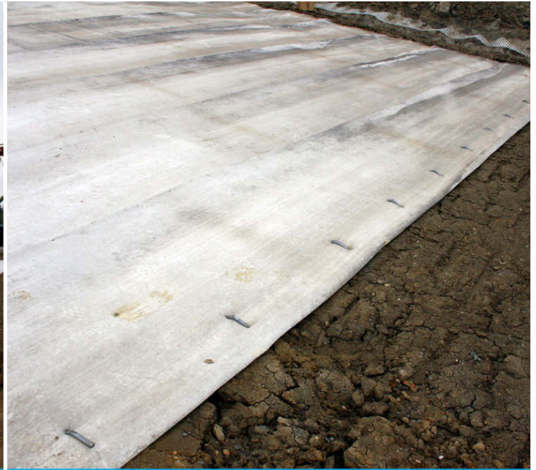
Metal fixings attaching the CC8™ to the clay substrate
