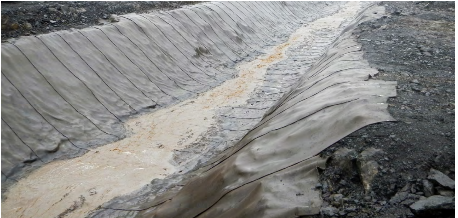
Completed lined ditch channel
