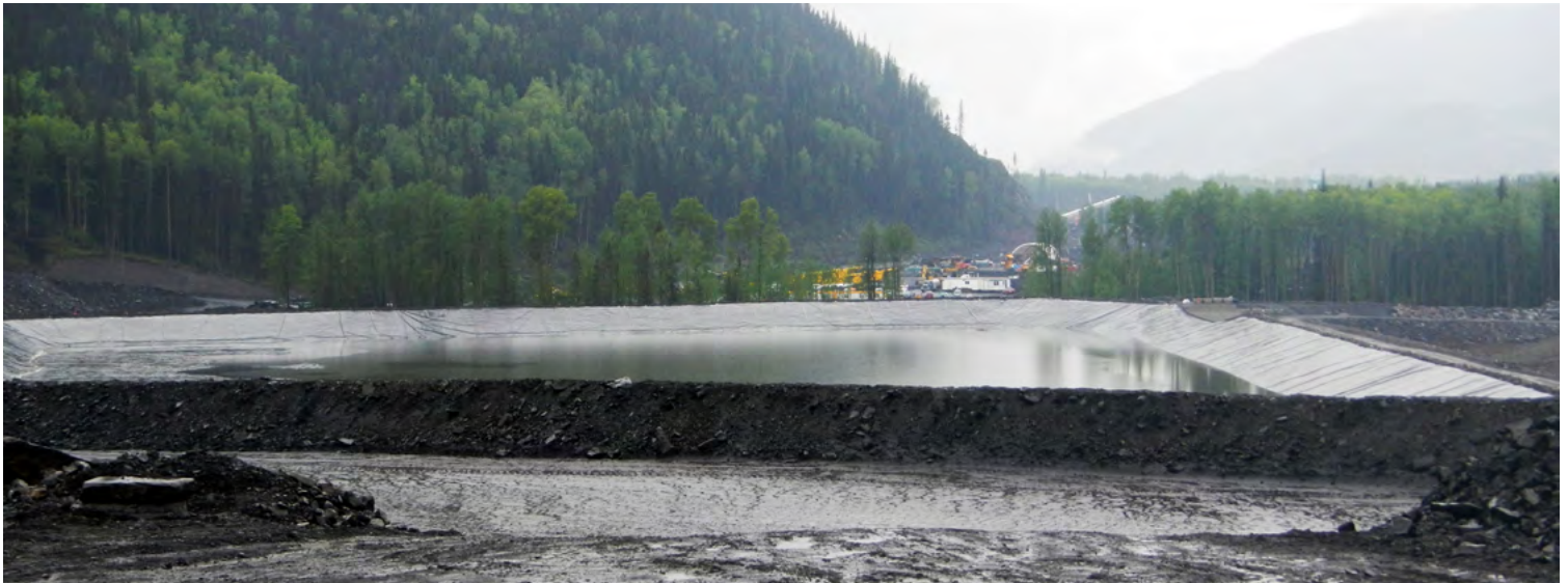
Large settling pond collecting effluent from nearby Willow Creek coal mine, British Columbia, Canada
