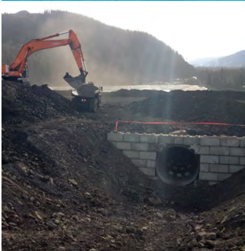
Excavating the sump and constructing the culvert
