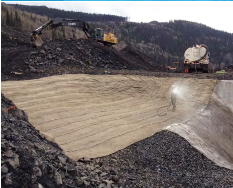
Swale was formed on the north ridge of the ditch at a nearby tree line to collect surface rainfall from an adjacent hillside.
