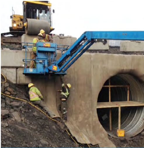
Lining the culvert with CC8
