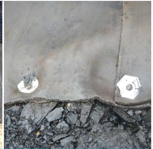
6" steel anchor nails with 1" hex head washers
