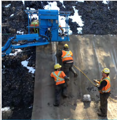
Applying Sikaflex beading to joints
