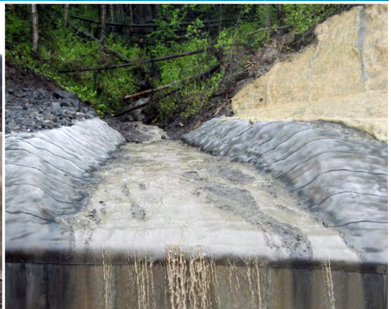
Swale was formed on the north ridge of the ditch at a nearby tree line to collect surface rainfall from an adjacent hillside.
