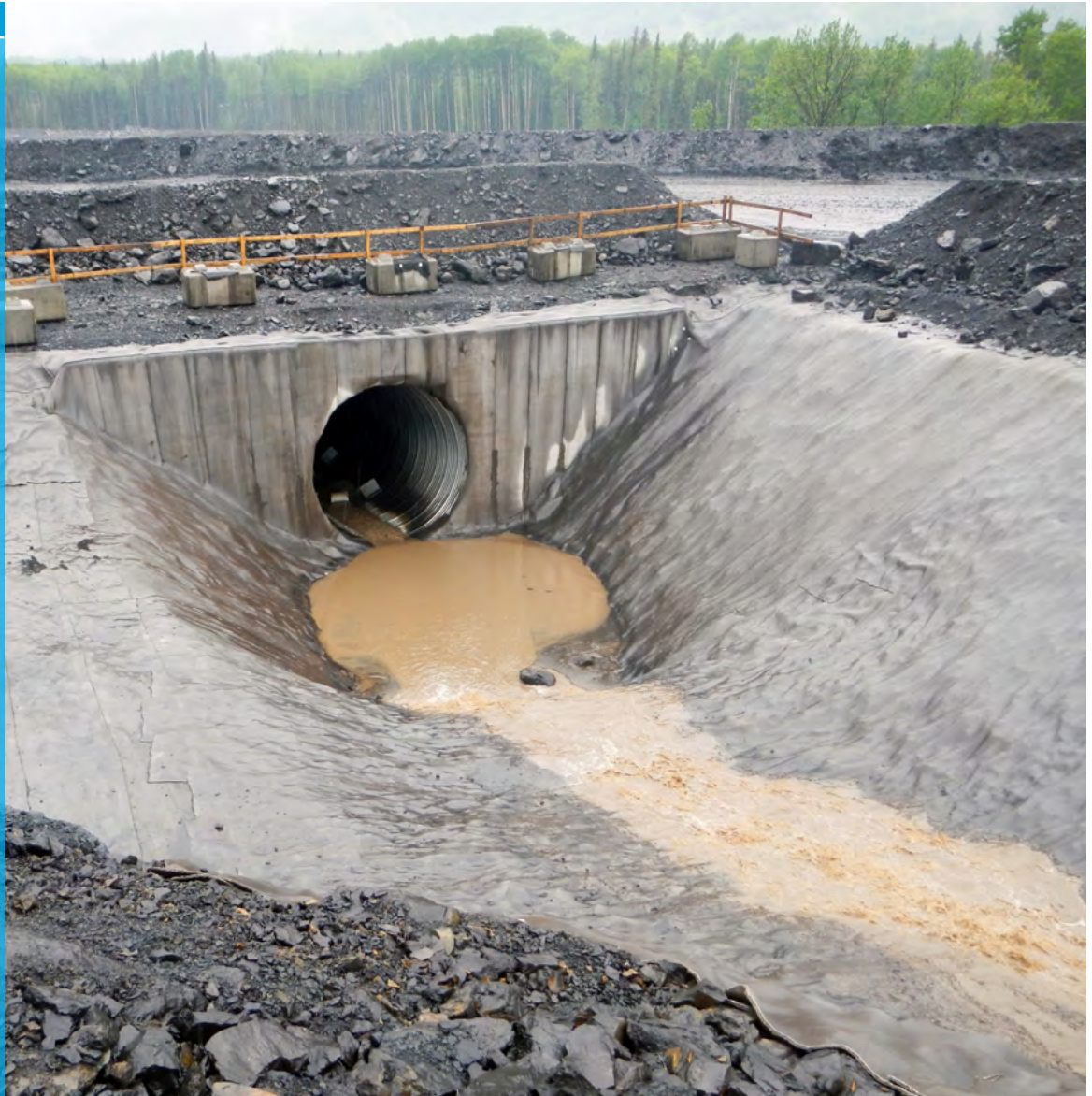
Completed lined ditch channel and culvert.
