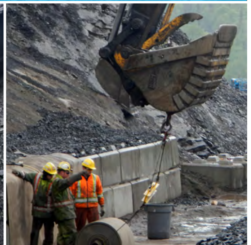
Using plant to unroll CC bulk rolls across channel
