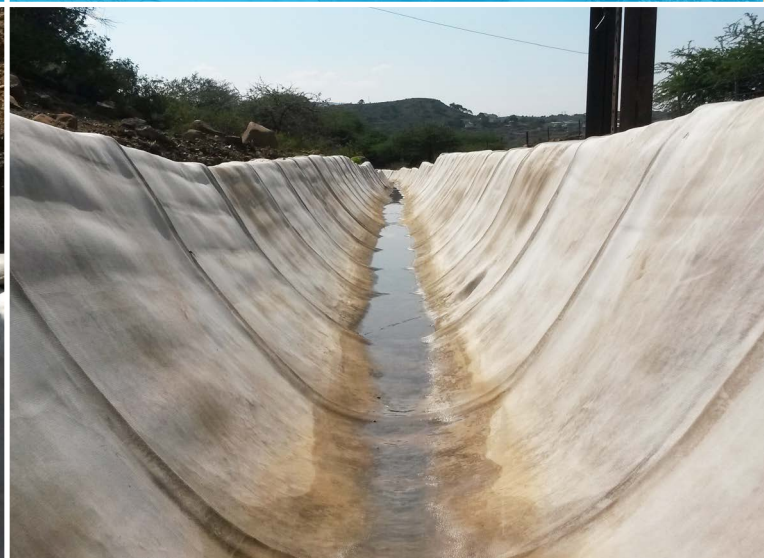
The completed ditch
