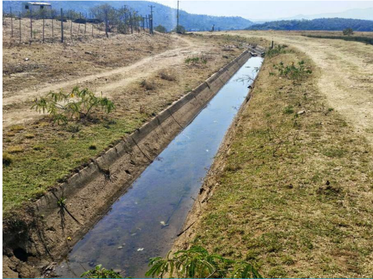
Site before works began
