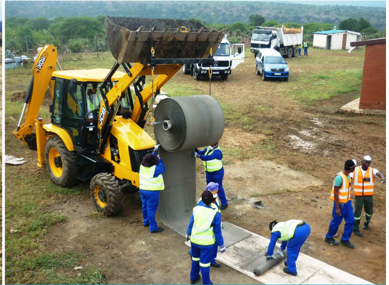
Dispensing the bulk roll for on-site batching
