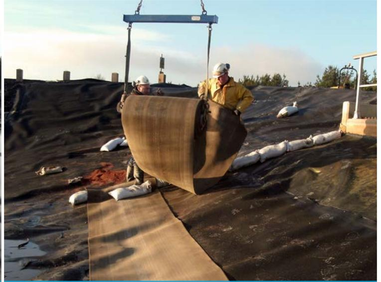
CC bulk rolls deployed from excavator using spreader beam
