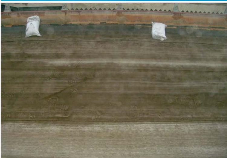
Hydration achieved by flooding adjacent pond, allowing it to spill over CC
