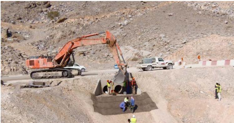
CC13™ batched rolls being craned into position from road access
