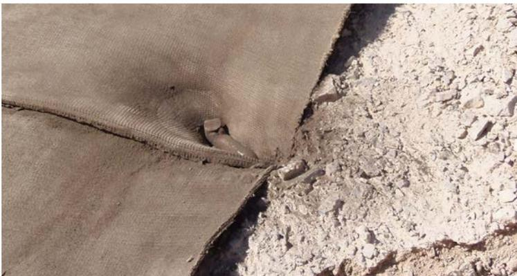
CC layer edges were fixed with ground pegs at overlapping joints
