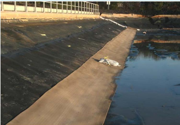
First layer of CC cut to length on site and fixed with CT1 adhesive
