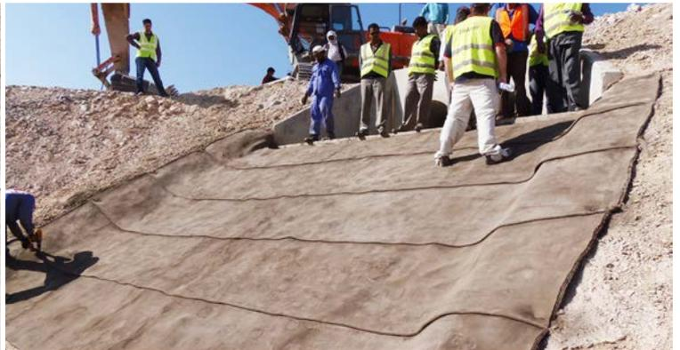
5 CC layers were installed in total
