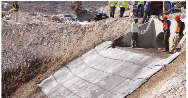
Once installed, the CC layers were hydrated from a bowser
