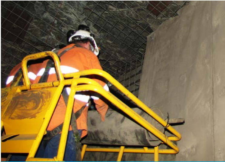
CC loaded onto the elevated work platform
