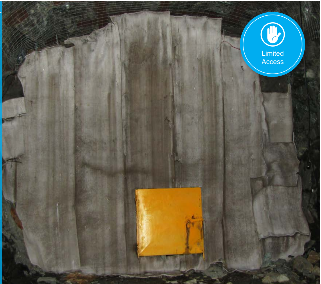
Finished vent wall
