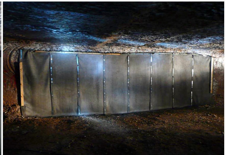
Completed vent wall closure using CC
