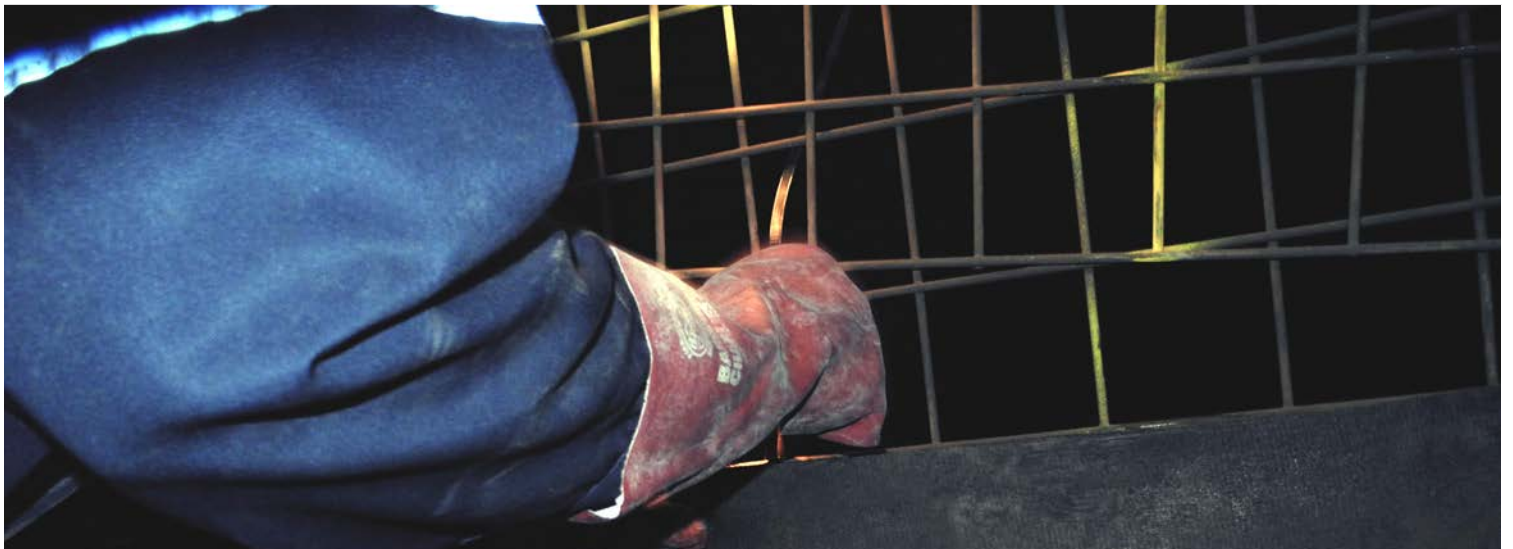
Attaching CC to the wire frame using 8mm gauge industrial cable ties
