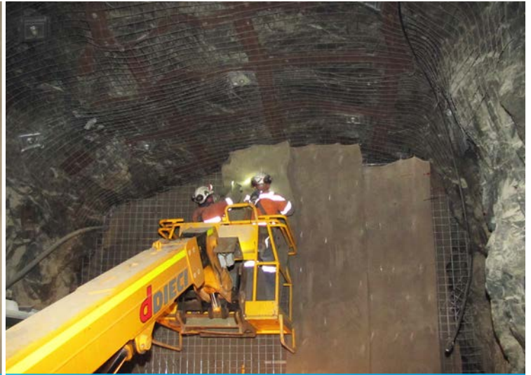
CC unrolled down the mesh
