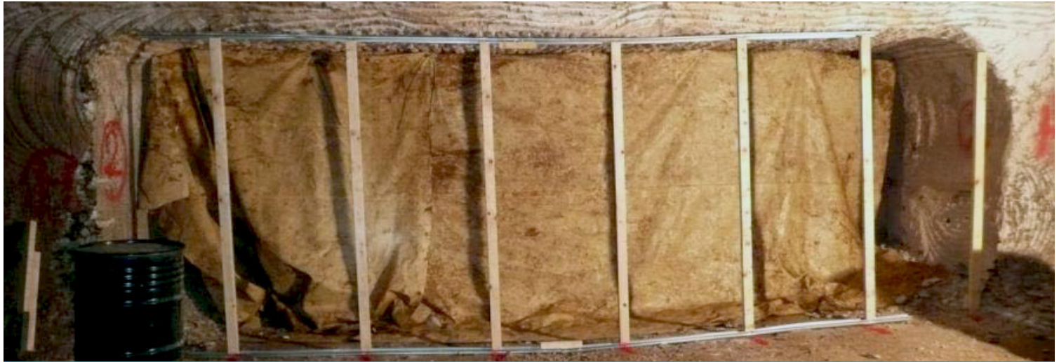
Frame created using British Gypsum branded aluminium stud wall system
