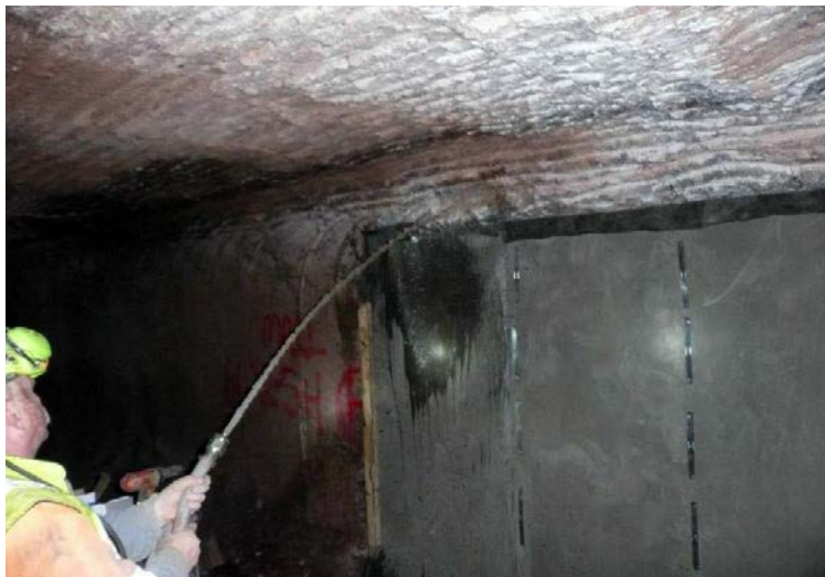
CC hydrated using on-site equipment
