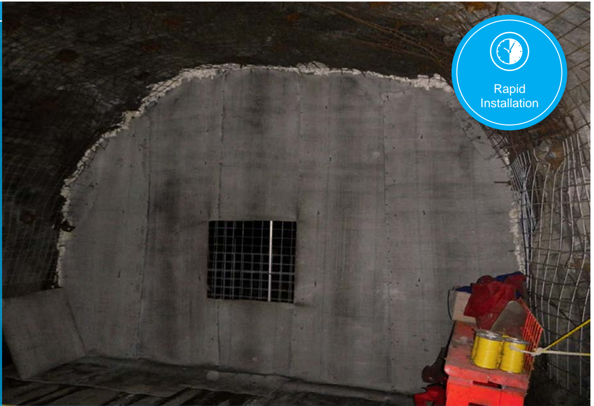
Completed vent wall closure
