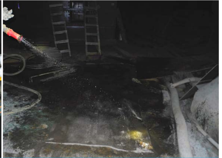
CC undergoing hydration prior to installation
