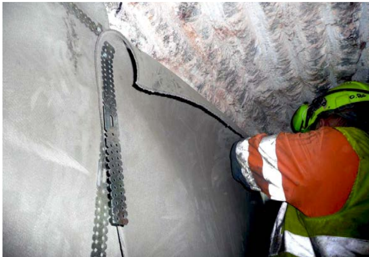
CC cut to size, held in place and screwed to frame
