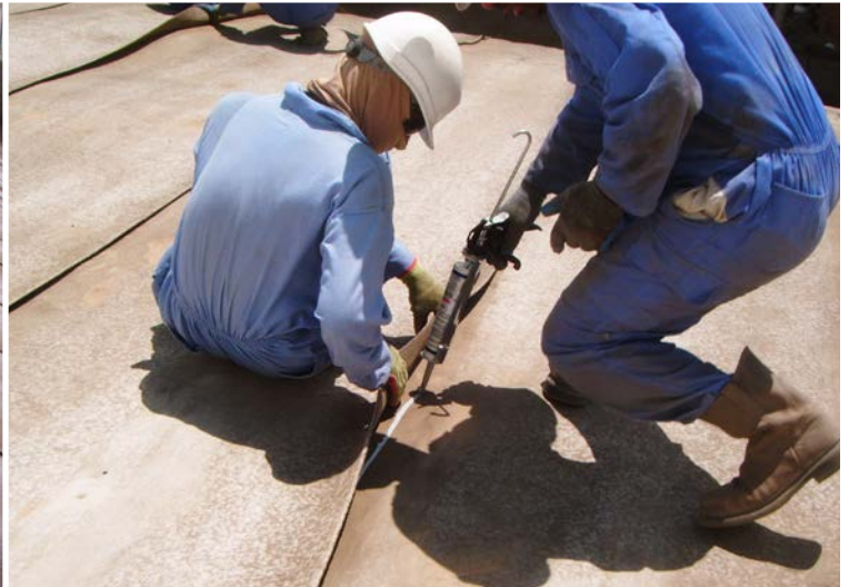
CT1 sealant being applied
