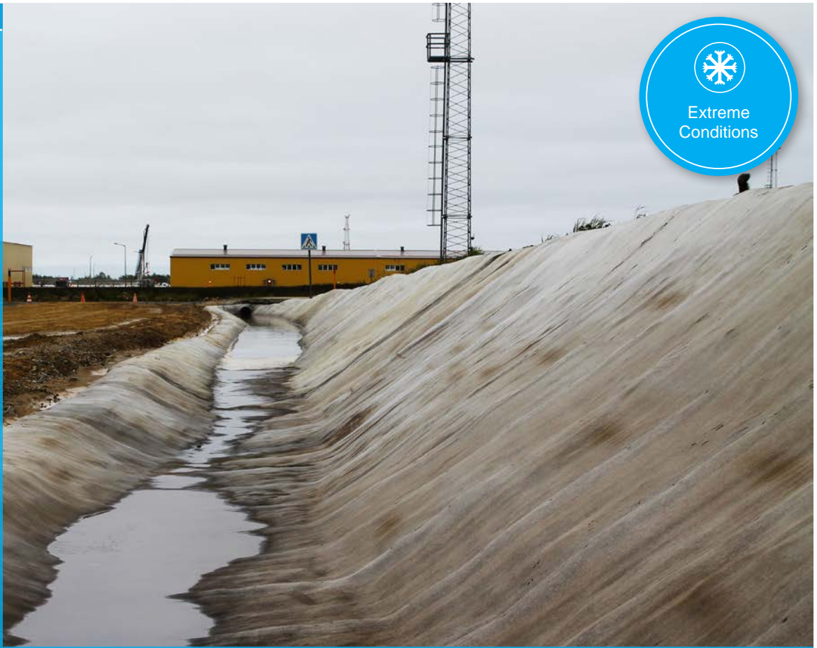
Completed section ditch lined with CC8™
