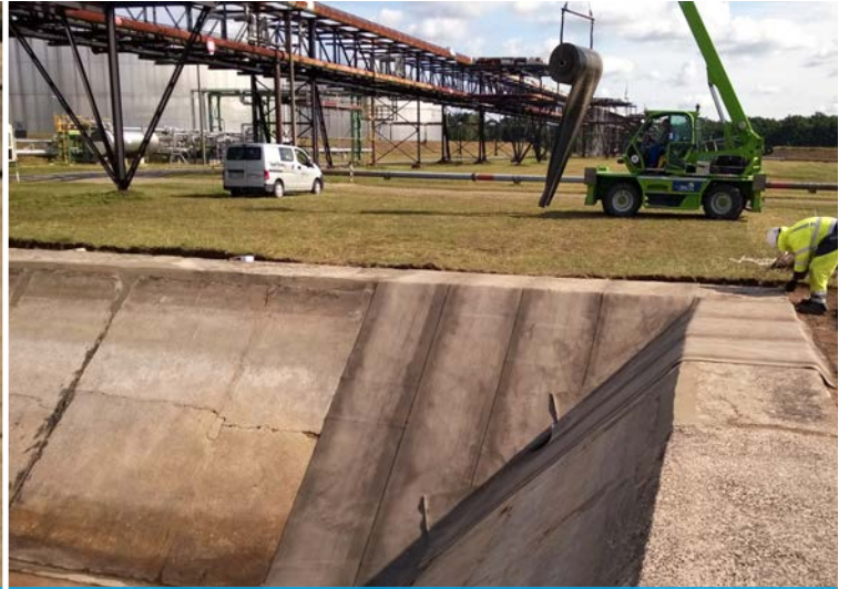
Batching on the flat and a corner detail
