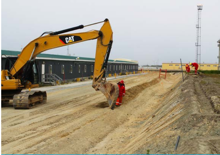
The ditch was excavated and graded to profile
