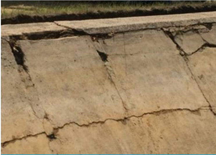
Site before works began
