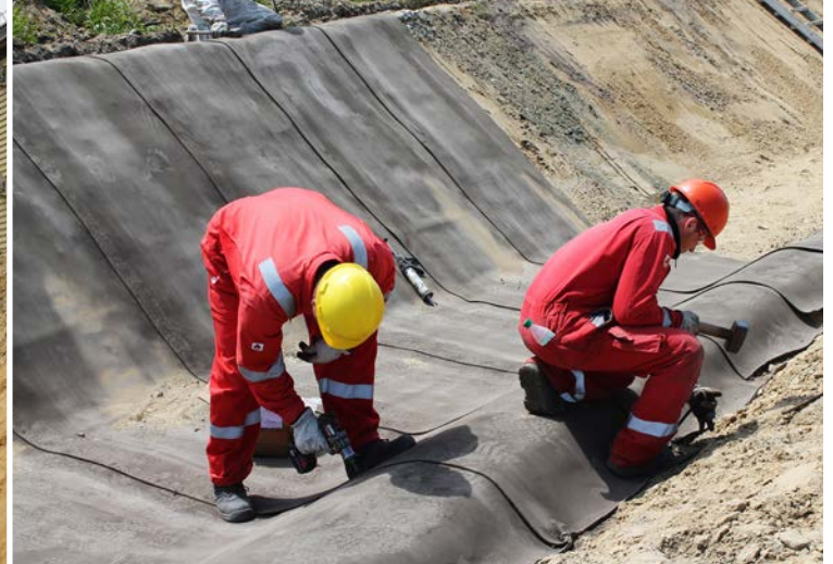
CC8™ sealed, screwed and fixed to the substrate with ground pegs
