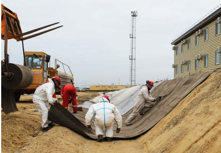
Unset CC8™ cut to length, avoiding wastage
