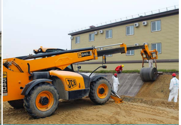
CC8™ bulk rolls were unrolled across the ditch and into anchor trenches
