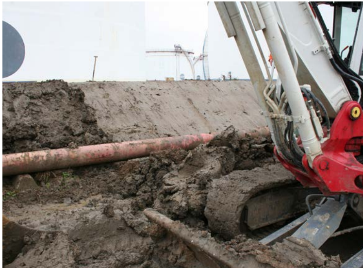
Prepare / grade clay bund to desired profile and height
