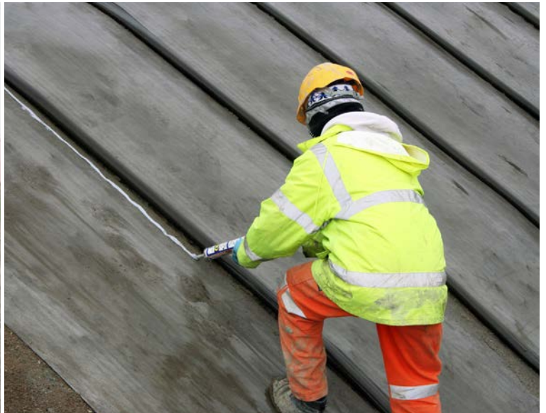
Adhesive sealing of 100mm overlapped joints using CT1
