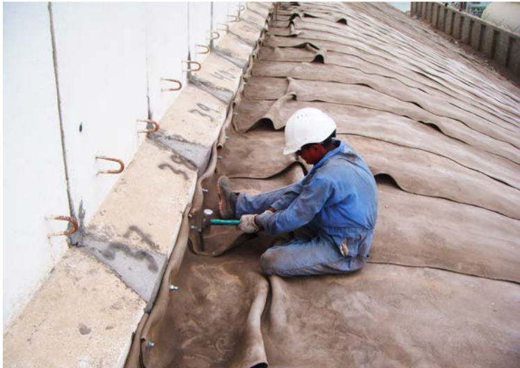
Masonry fixings and ground pegs
