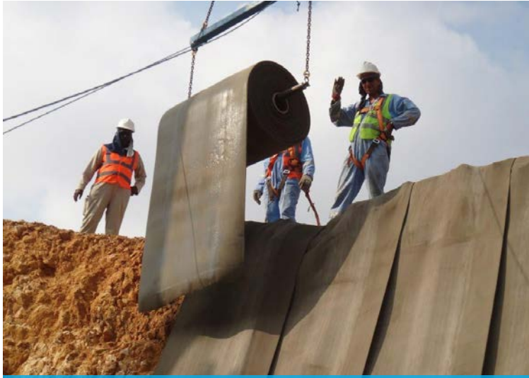
CC being lifted into position
