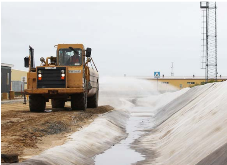
Hydration with a pressure hose from a 7000 litre bowser
