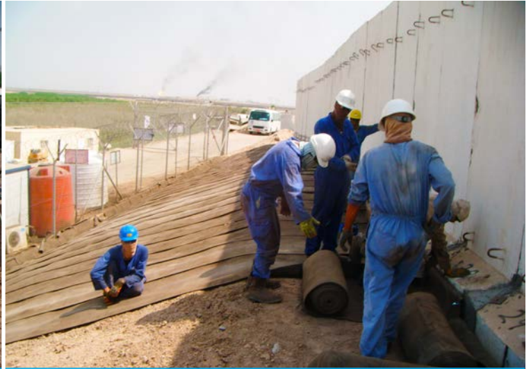
CC8™ lengths unrolled down the slope
