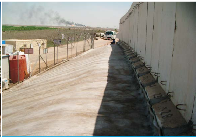
The finished slope
