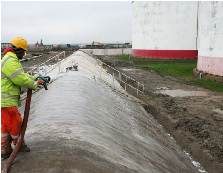
Hydration of CC from on site mains water supply
