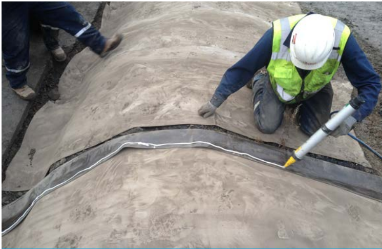
Sealing the overlap with CT1 Sika1-A sealant
