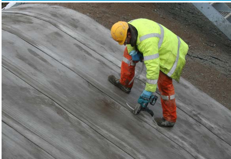
Joining of adjacent layers using 30mm autofed screws
