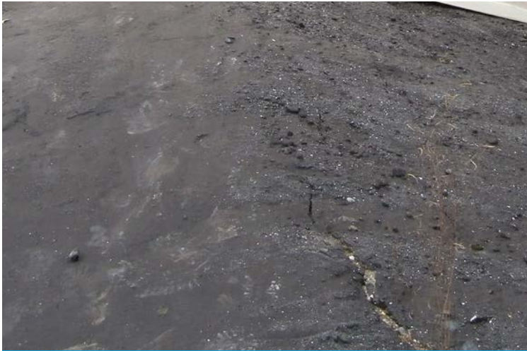
Cracked asphalt
