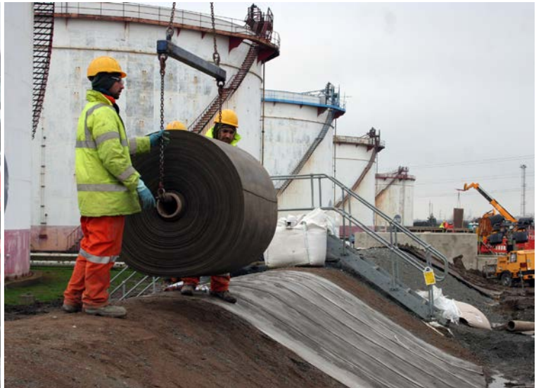
Transverse layup of bulk roll CC5™ from spreader beam
