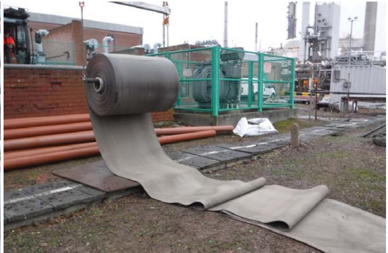
Dispensing of bulk roll CC8 via spreader beam.
