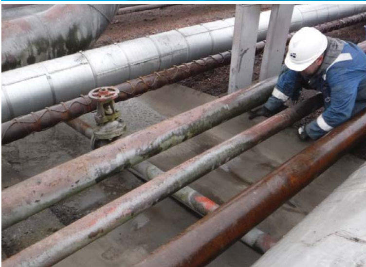
Adjusting position to create 100mm overlaps prior to screwing joint.
