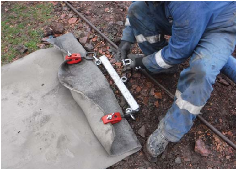
Attachment of low profile pulling jig.
