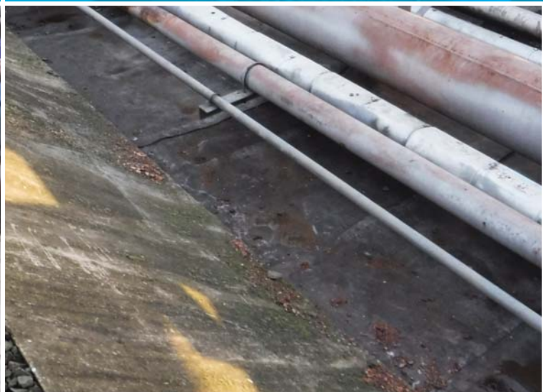
CC8 terminations to existing concrete infrastructure.
