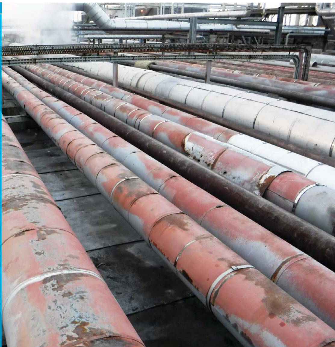
Completed CC lined pipe track.
