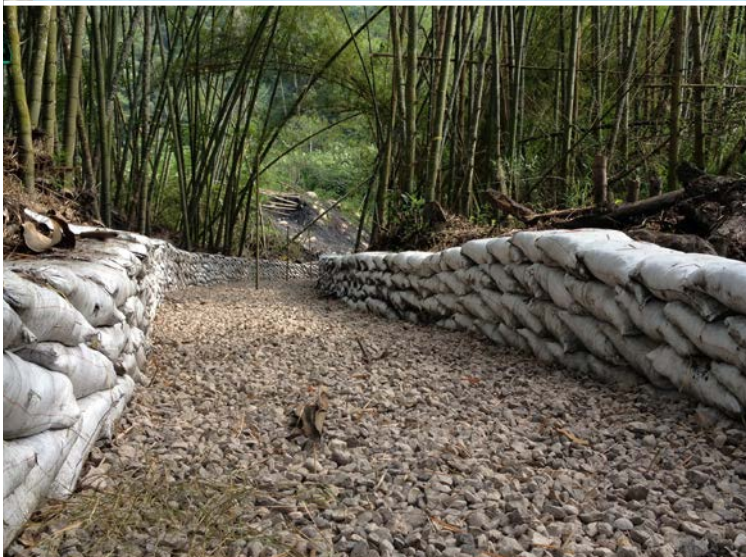
Ditch profile prior to lining with CC
