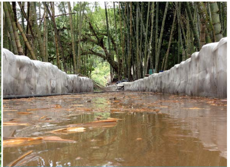
Completed CC lined ditch with redirected water flow
