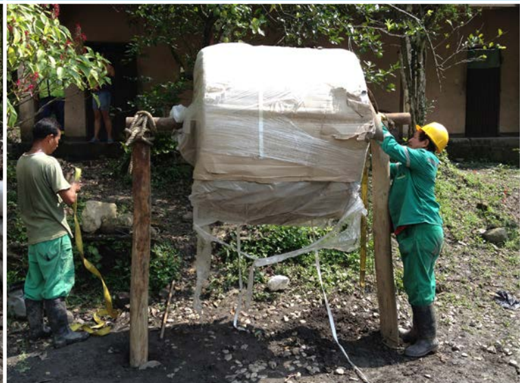
CC dispensed from a bulk roll on site before being cut to length
