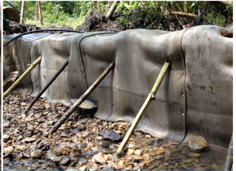
Wooden beams were used to close voids immediately after hydration
