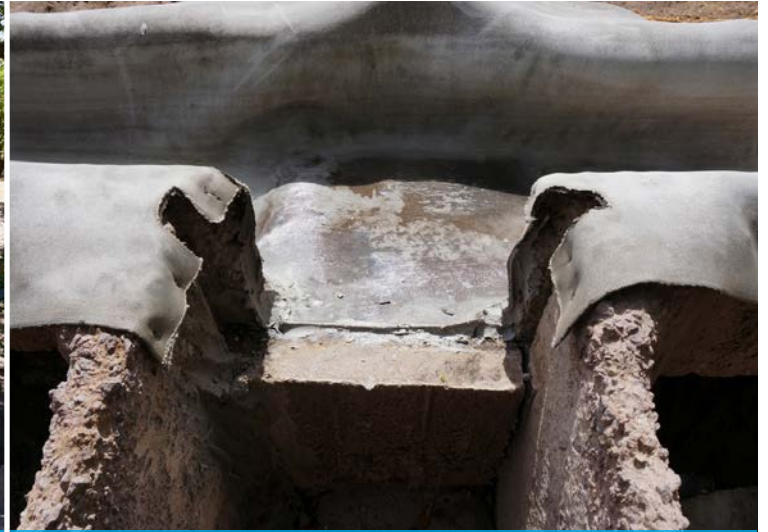
An epoxy grout joint to allow for the steel doors
