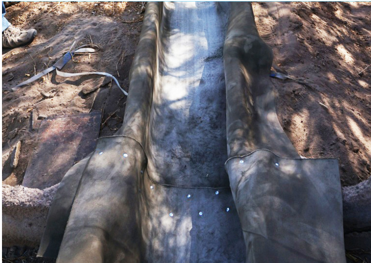
Overlapped and screwed joint
