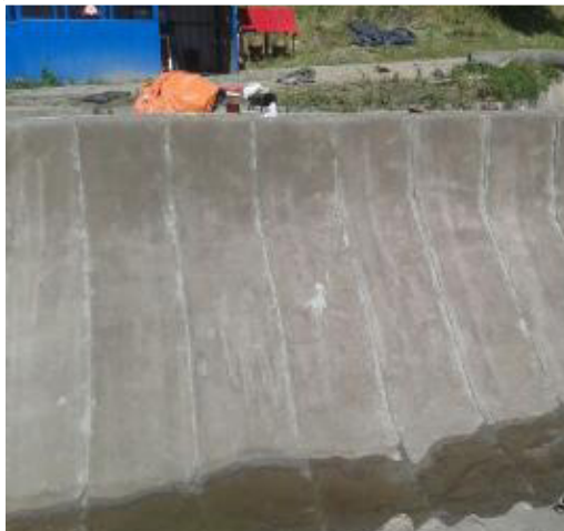
Lined concrete reservoir with sealed joints
