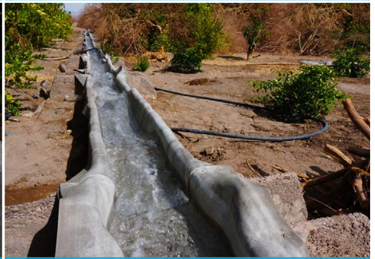
The finished ditch
