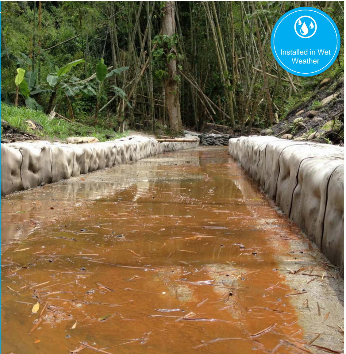
Completed CC lined ditch section, Nocaima, Cundinamarca, Colombia
