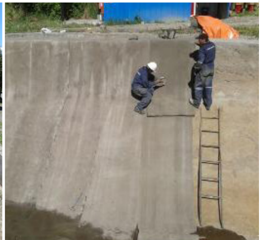
Fixing CC to the existing concrete substructure
