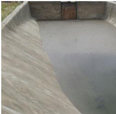
Refilling the basin to hydrate the CC
