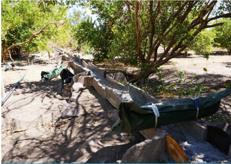
A batched roll of CC5™ and the broken ditch
