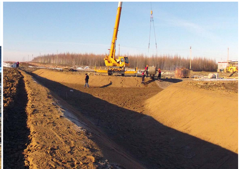
CC mounted onto a spreader beam and hung from a crane
