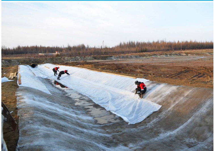
Protecting the CC with plastic sheeting
