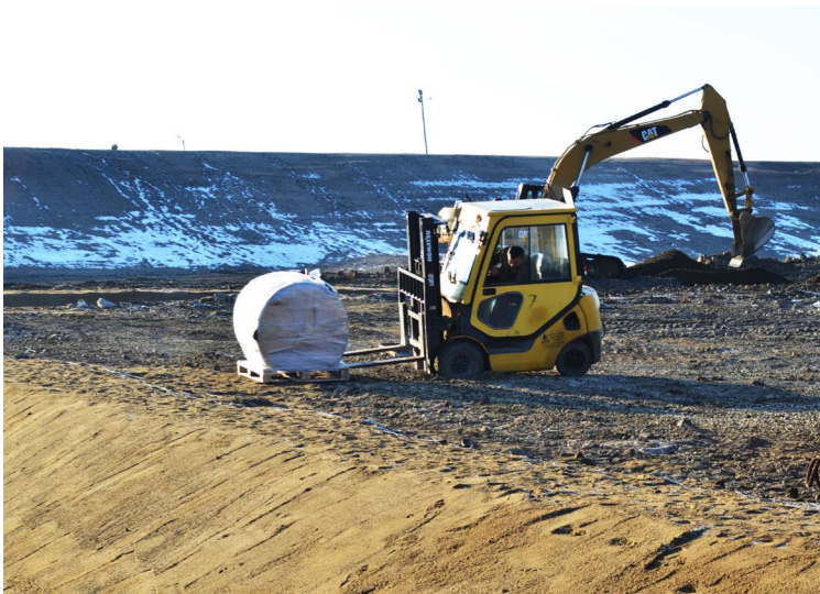
Bulk roll of CC13™ being delivered to site
