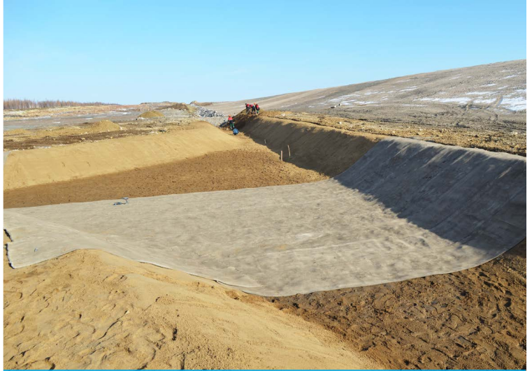
CC unrolled across the ditch
