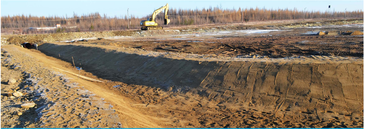
The excavated ditch
