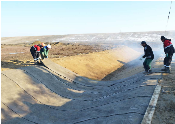
Overlapping the CC by 100mm
